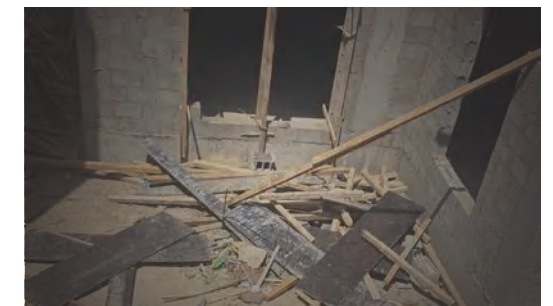
Timber Formwork on Site
