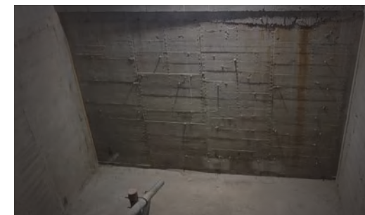
Timber Formwork Forming Effect
